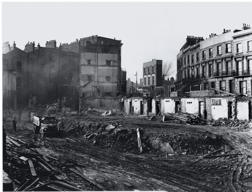
Clarendon Crescent, Paddington, under demolition
